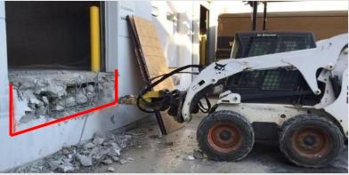
Unknown hazards exposed during building floor demolition.
