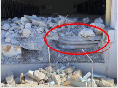
Electrical conduit discovered during construction.
